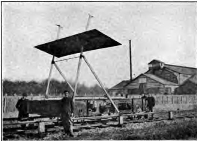
FIG. 2. FIRST PLATFORM EQUIPPED FOR TRIAL AT AEROTECHNIC INSTITUTE OF SAINT-CYR
